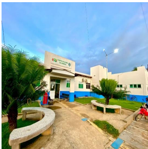
Figura 205 - Vista do Hospital Regional de Buritis, 2024
