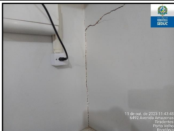
Trinca vertical e horizontal
