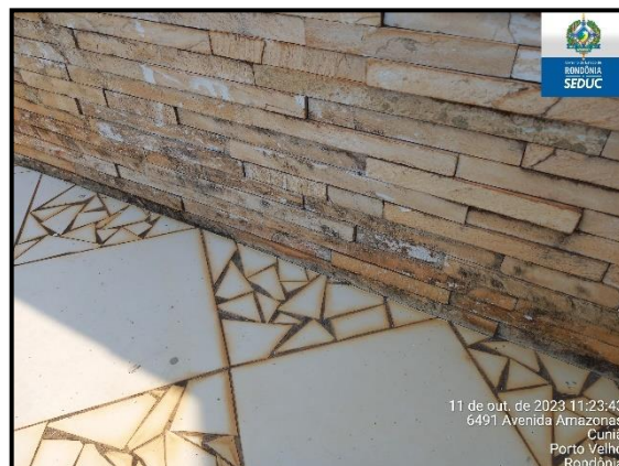
Fissura filetes fachada
